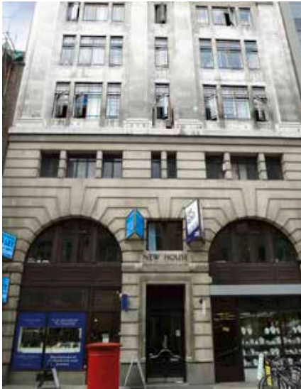
KERN UK Ltd., New House, Rooms 45/46, 67/68 Hatton Garden
